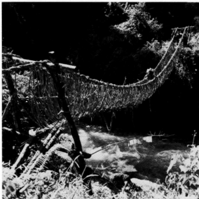
Fig. 15. A primitive hanging bridge in the north-eastern Bhutan Himalaya. This bridge is built in a primitive way, only by liana and bamboo, a system over 2000 years old. (Fot. A. Gansser).
